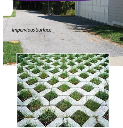
Permeable Pavers Photos by Matt Kofroth, LCCD
